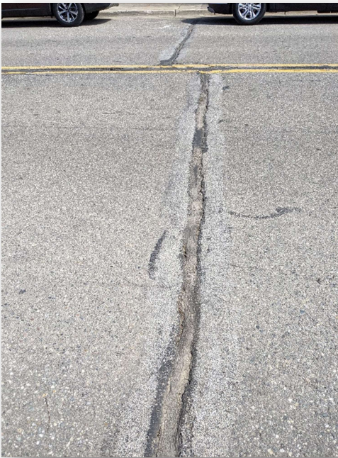
Photo 2 - Transverse Cracking
